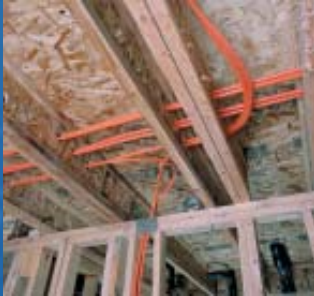
Running flexible piping through walls, floors, and ceilings costs less and takes less time than installing forced-air heating ducts.
